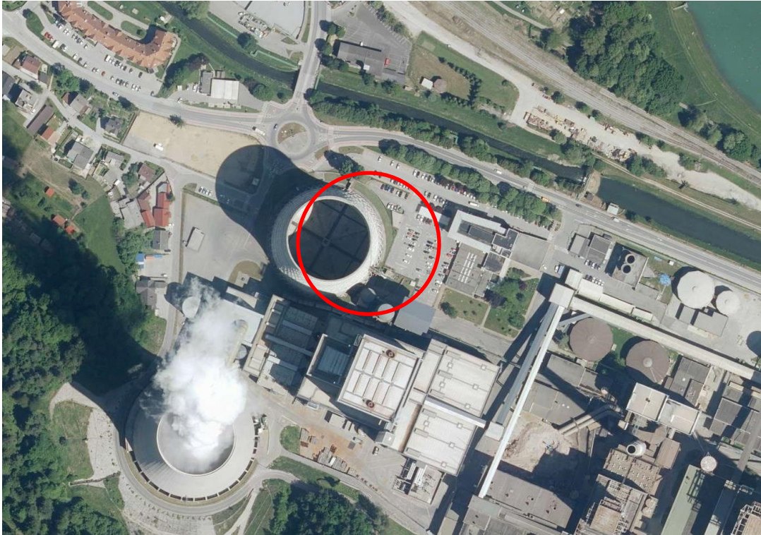
Figure 1: Areal photo of the area with the Unit 4 Cooling tower
